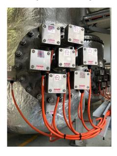
Each heater is controlled with Solid State relays, effectively controlling the heat input and resulting batch temperature rise.
