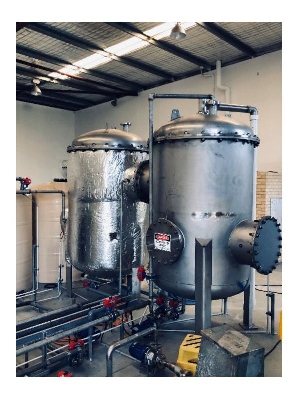
To reduce energy consumption, the plant is designed with a post run heat recovery circuit including a plate heat exchanger. The plate exchanger is used to recover heat from the kettle waste, being used to preheat the temperature of the next batch. The new batch is heated to approximately 45-50 degrees C when entering the pre heater, where it is further heated to 60-65 degrees C. All hot equipment and components are fully insulated for personnel protection and to reduce energy loss.
