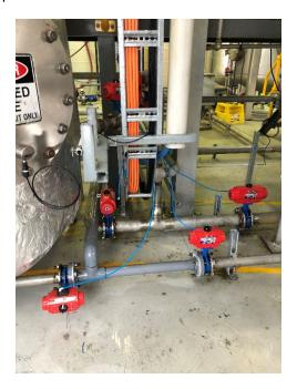
The plant could be further expanded with the installation of a third kettle. The existing piping arrangement has been configured to facilitate the third kettle without significant modification.
