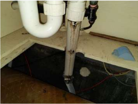
Ref # 13.8 - Leaking rear head sink
