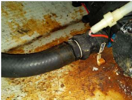
Ref # 13.4 - Plumbing system condition ( no hose clamp)
