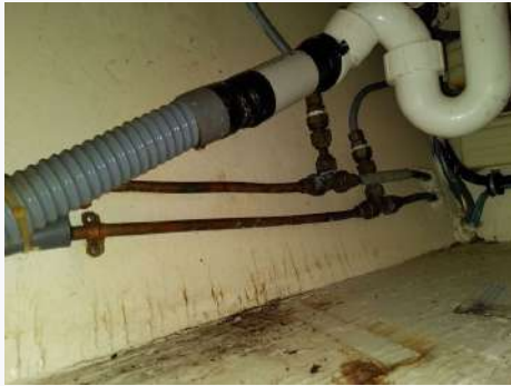
Ref # 13.8 - Leaking starboard head sink
