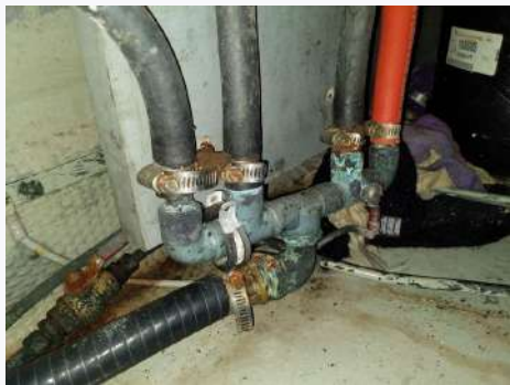
Ref # 15.3 - Air Conditioner intake manifold
